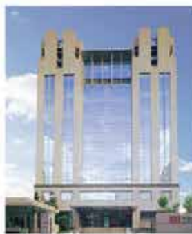
MEAN WELL GUANGZHOU TIANHE R&D CENTER
